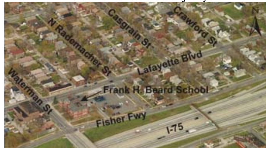
Figure 3.1-4 Aerial View of Frank H. Beard School Detroit River International Crossing Study
