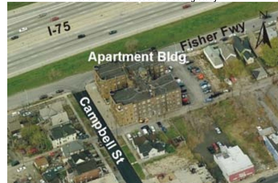
Figure 3.1-6 Aerial View of Berwalt Manor Apartment Building Detroit River International Crossing Study
