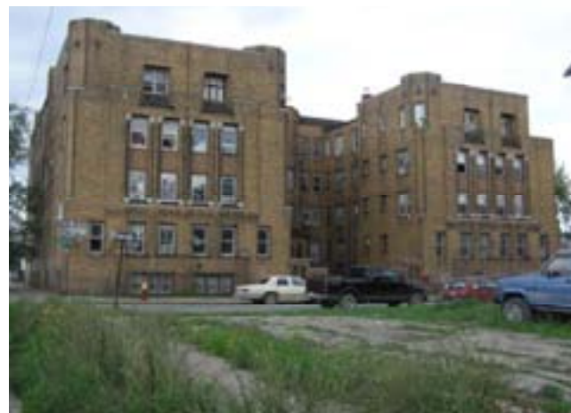
Figure 4.3-1 Berwalt Manor Building
